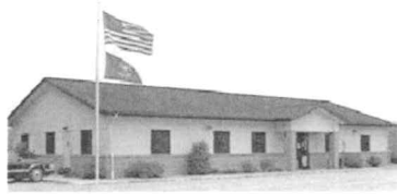
Porter Township Administration Offices
